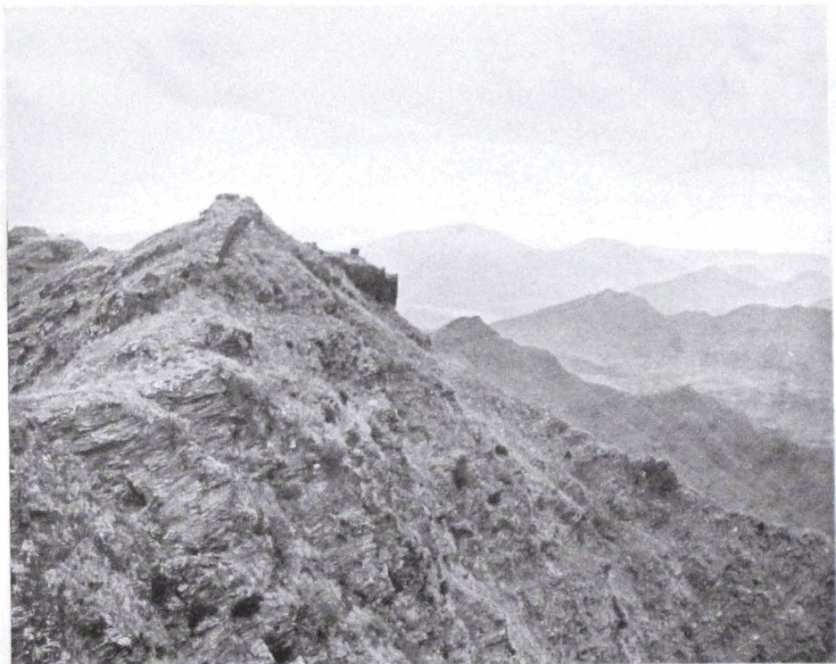
27. VIEW ALONG FORTIFIED HILL CREST, RĀJA GIRĀ'S CASTLE, UḍE-GRĀM.
