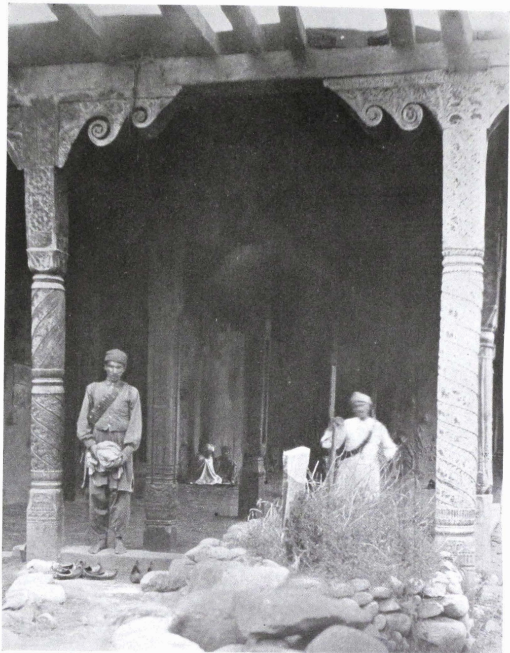
53. WOODEN PILLARS WITH CARVINGS IN LOGGIA OF PRINCIPAL MOSQUE, BRANIĀL.
