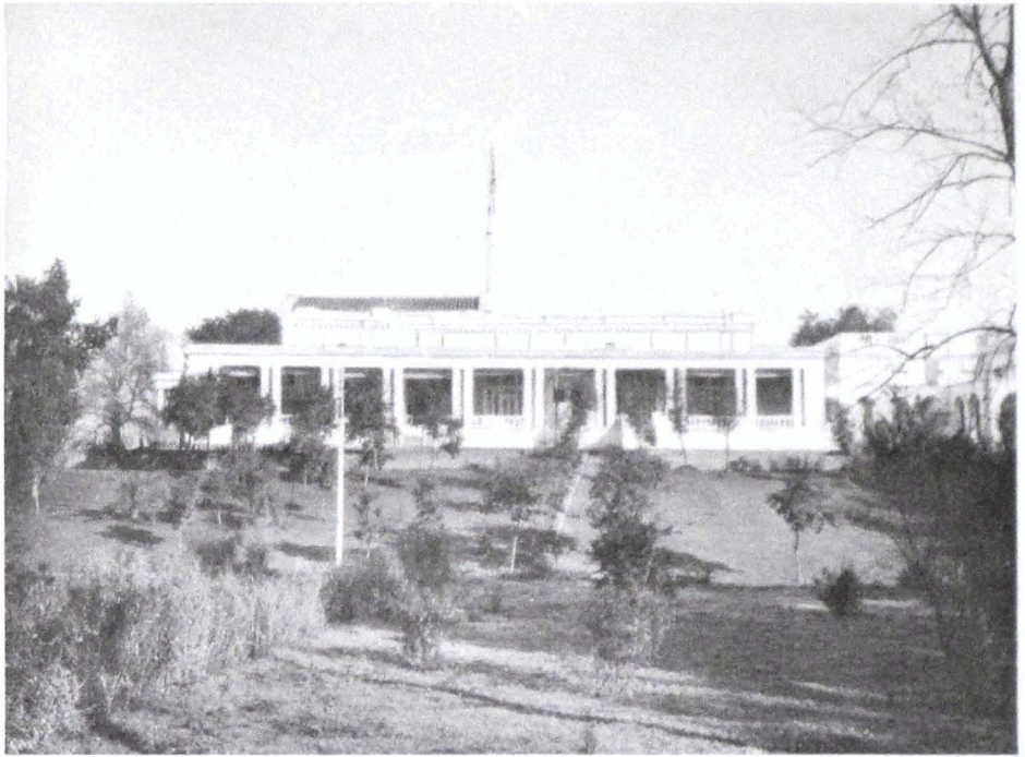
2. GOVERNMENT HOUSE, PESHAWAR. Residence of the Chief Commissioner, North-West Frontier Province.
